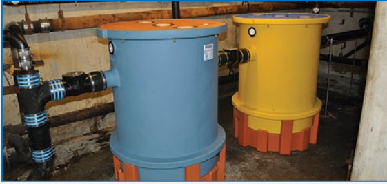
A Solids Separator installed ahead of a Trappzilla GI servicing the food prep area of a national grocery chain.
