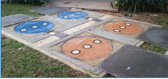
Two TSS-95 Solids Separators in front of two TZ-600 Grease Interceptors servicing a large cafeteria in a high-rise office building.
