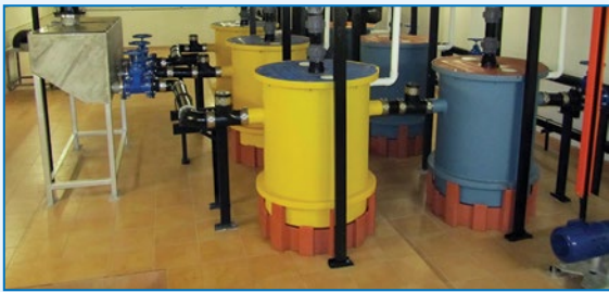
Trappzilla Grease Interceptors and Solids Separators servicing a Major International Hospital
