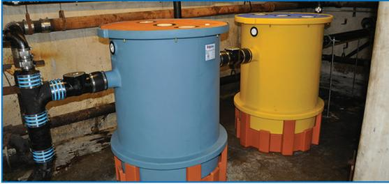
A Solids Separator installed ahead of a Trappzilla® GI for the food prep area of a national grocery chain.
